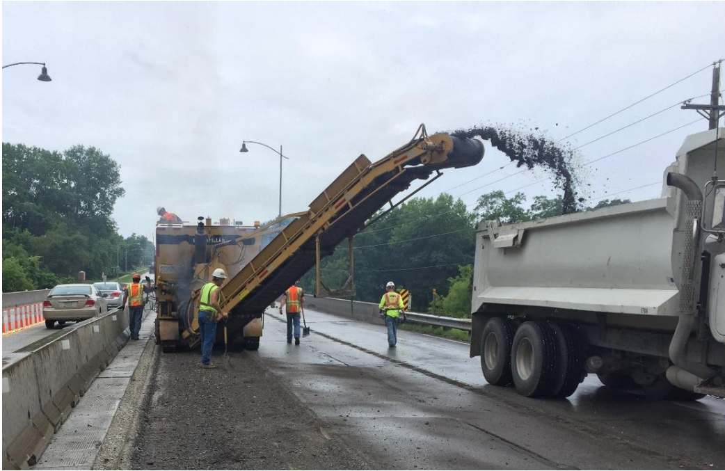
Figure 41. Milling machine removal of top layer of the deck
