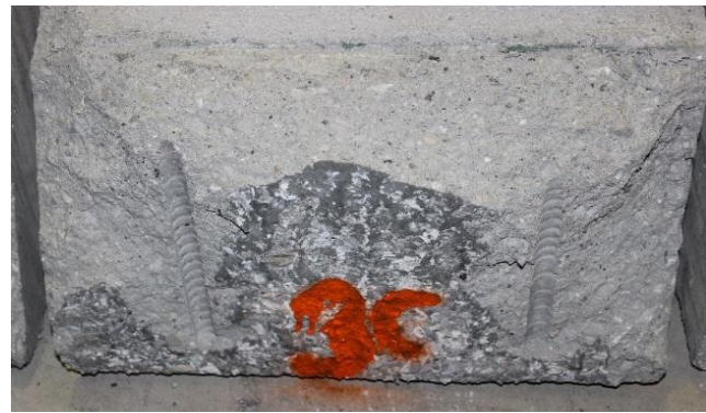
d) Bond interface (overlay concrete)
