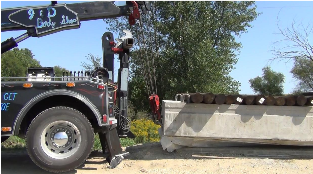
a) Beam lifted by tow truck
