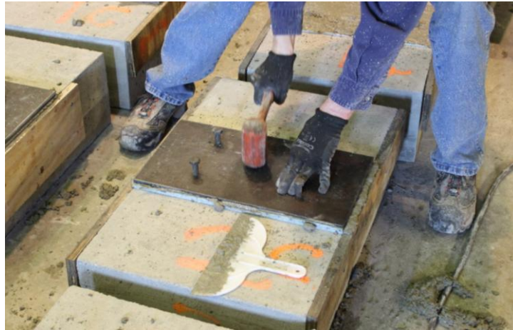
Figure 53. Tapping the steel plate to embed the shear studs on a pull-off test specimen
