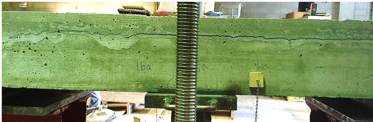
Figure 86. Case 1 positive bending flexural test specimen failure at concrete bond interface
