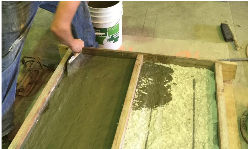
Figure 97. Application of grout to negative bending flexural test specimen
