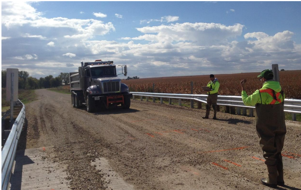
Figure 30. Carrying out the load test on the bridge
