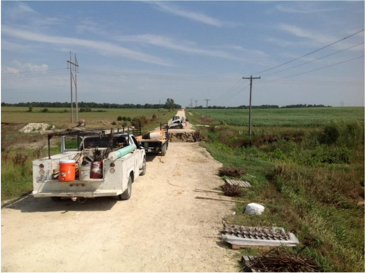
Figure 7. Construction job site
