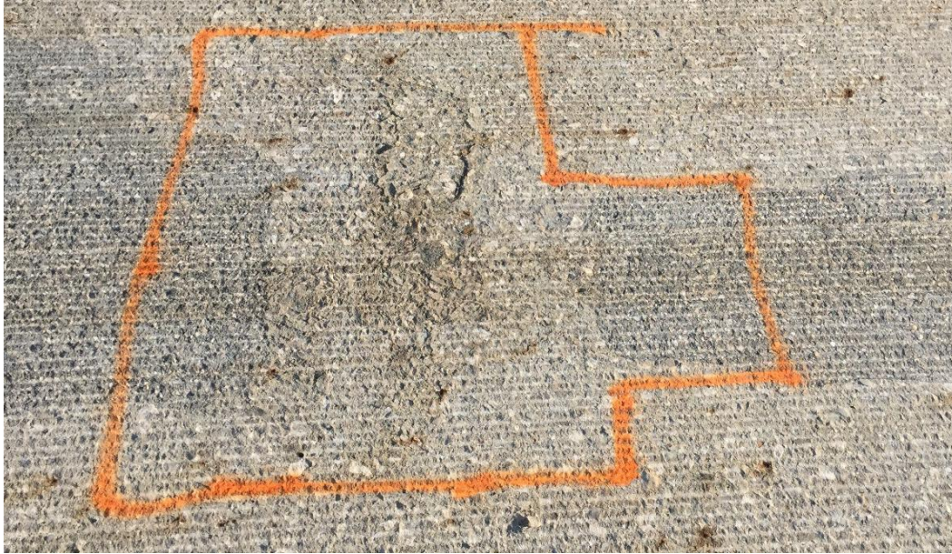
Figure 42. Area marked for more in-depth removal
