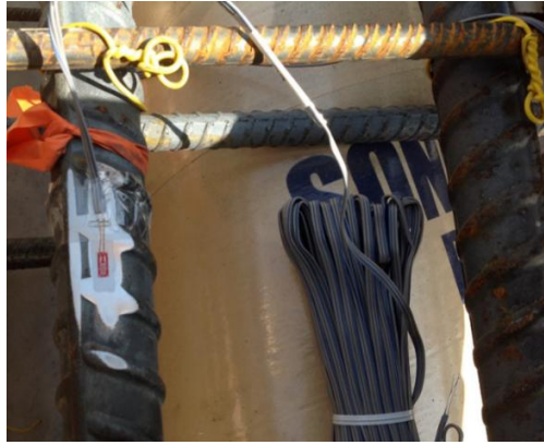
Figure 10. Gage installation on reinforcement
