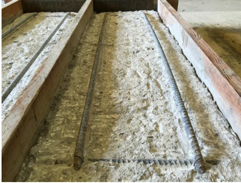
Figure 96. Negative bending flexural test specimen after concrete removal to required depth (Case 3)
