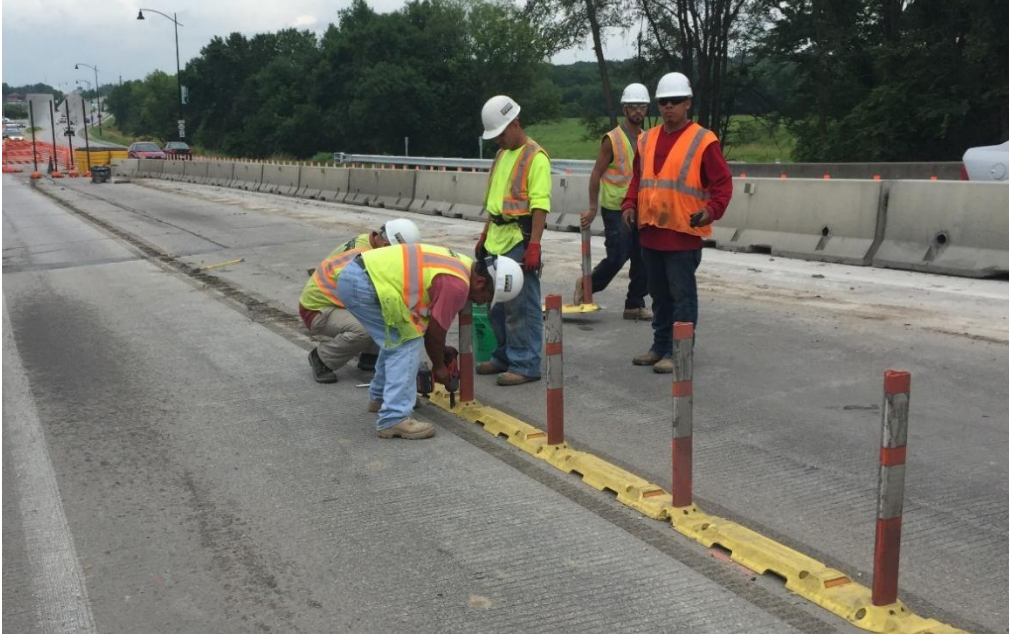
Figure 40. Temporary bollards being detached by workers
