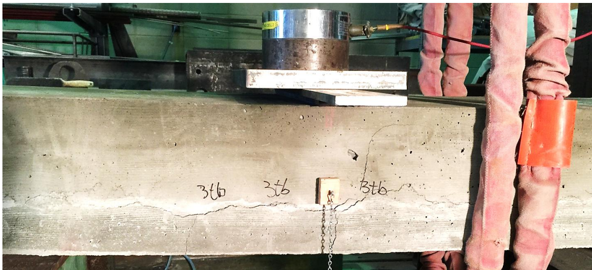
Figure 101. Case 3 negative bending flexural test specimen failure at concrete bond interface
