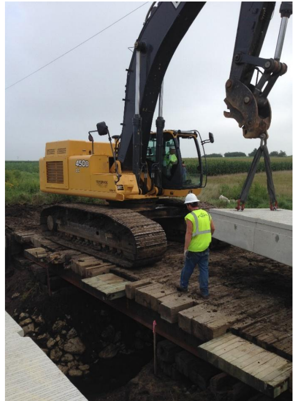
b) Beam move over the creek
