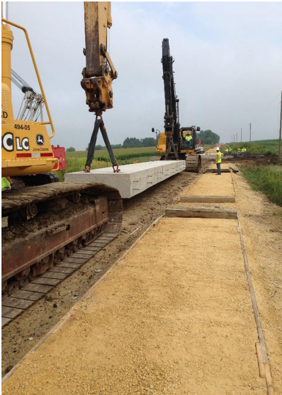
a) Beam lift
