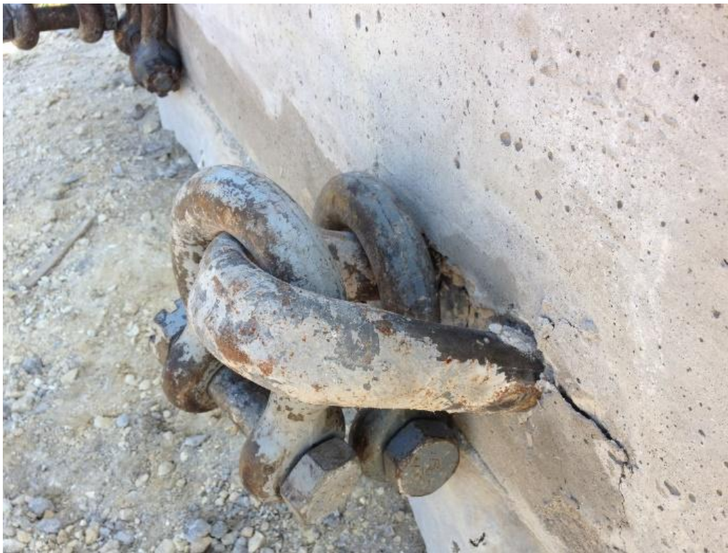
Figure 13. Horizontal pulling loops after lift
